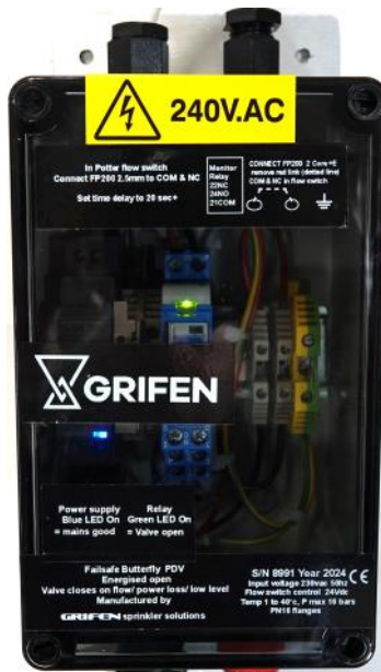
Control box with labels and LEDs
